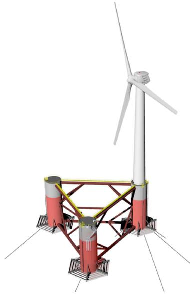
Figure 1.7: The WindFloat buoyancy-stabilized design
