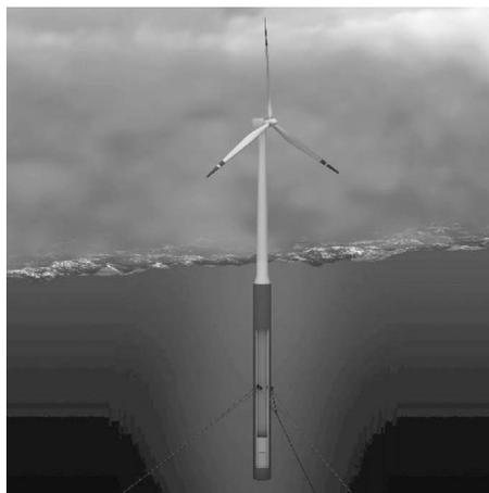
Figure 1.4: The Statfjord Hywind 2.3 MW ballast-stabilized prototype
