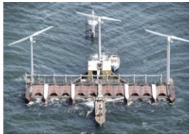
Figure 1.5: The Floating Power Plant Poseidon 3x11 kW prototype
